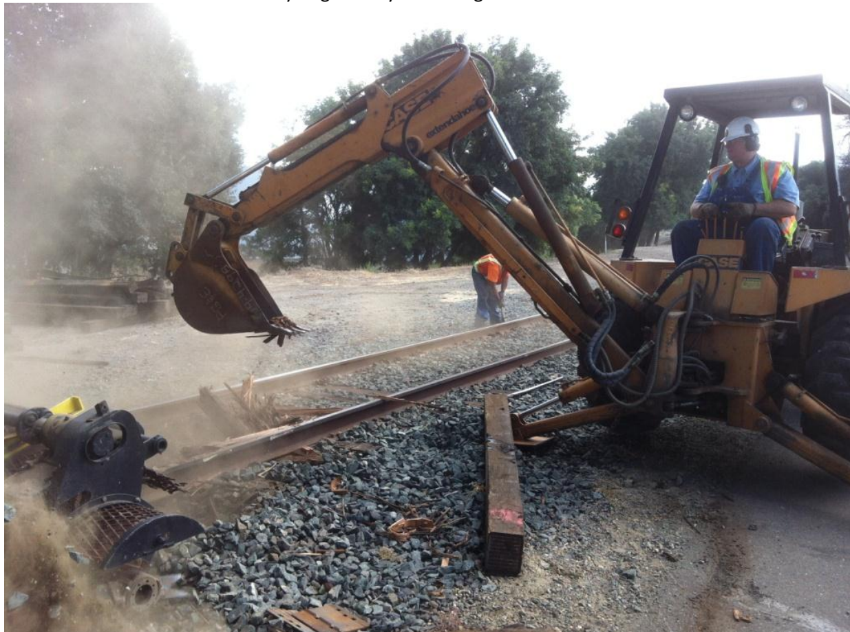
Chris digging out a splintering tie as the scarifer scarifies a tie crib
