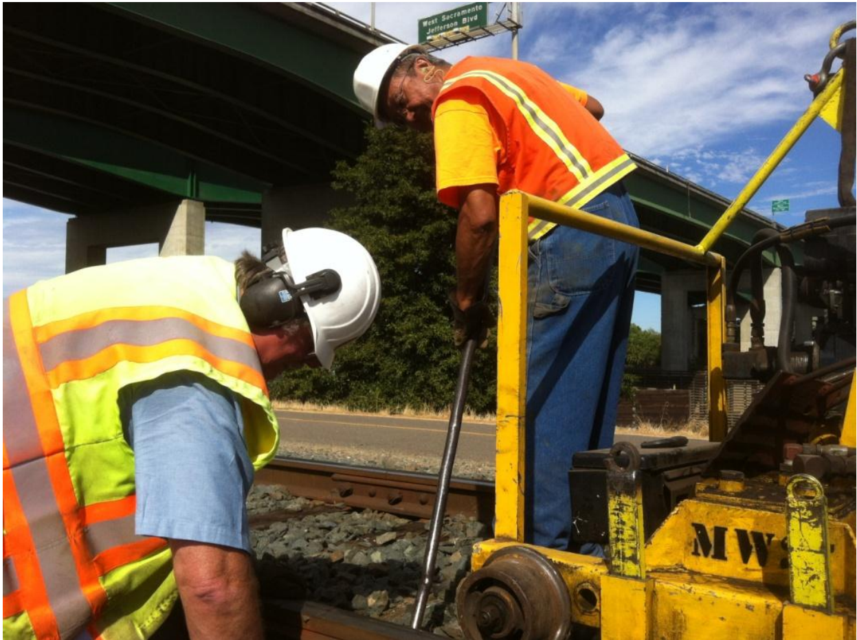
Chris and John pry out a tie plate
