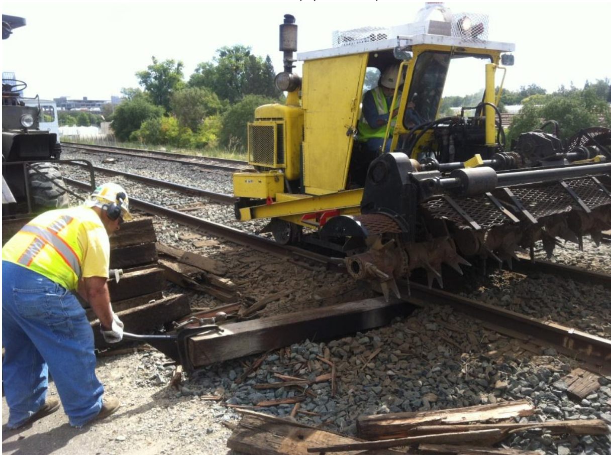
Alan working the scarifer/inserter as Mike F. uses the inserter function to insert a new tie
